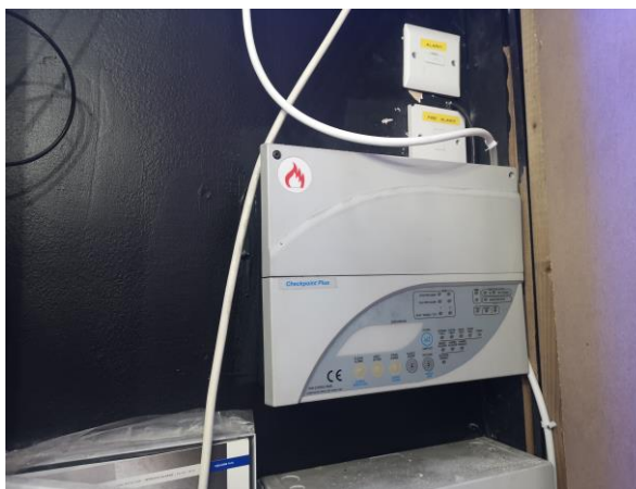
Fire control panel with no power
